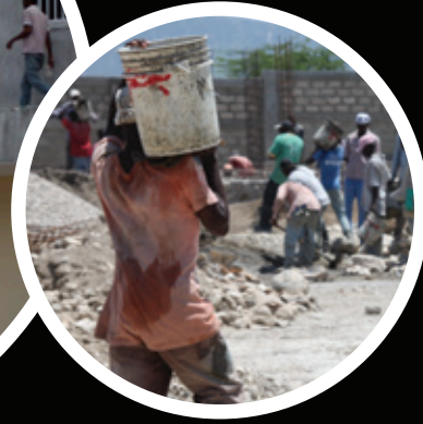
Construction continues at the Academy. Teams work around the clock to make sure school is open on time.
